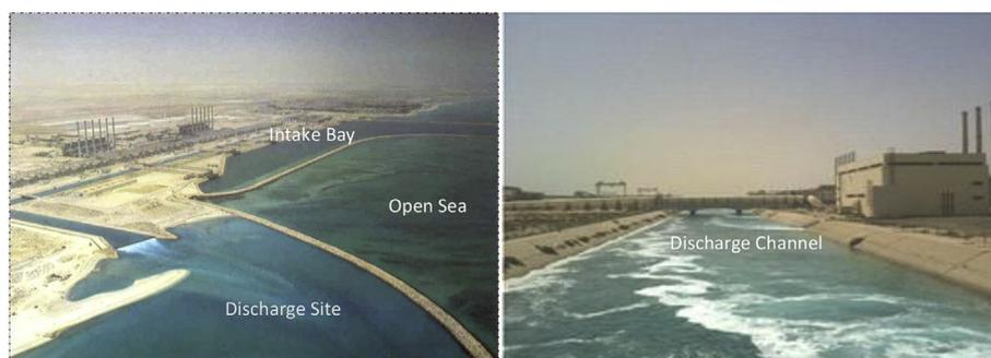
**Fig. 2.** General view of the intake and brine discharge system and coastal area of the Jubail desalination and power plants (left), and close view of the brine discharge channel (right).
