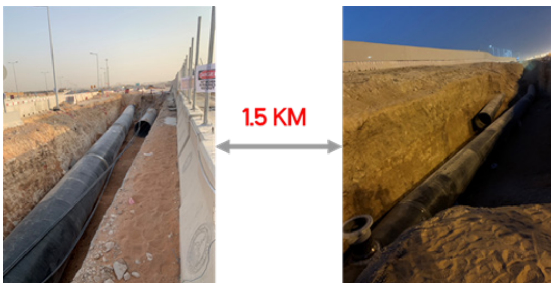
Figure 26 Inlet and Outlet of Inspected Underground Pipeline
